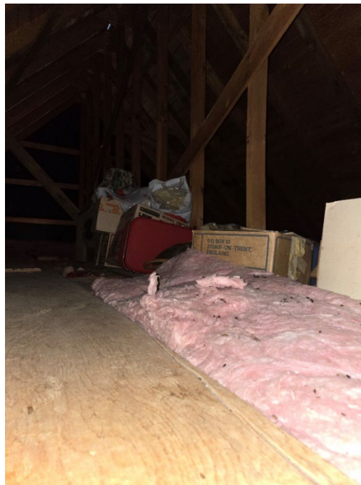
Picture 3: The attic contained fibreglass insulation.
