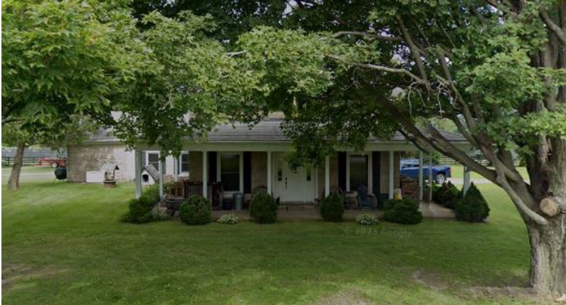
4303A Cove Road - The Joseph Green House - Built 1850 Lot 22 Concession 2 (?)
