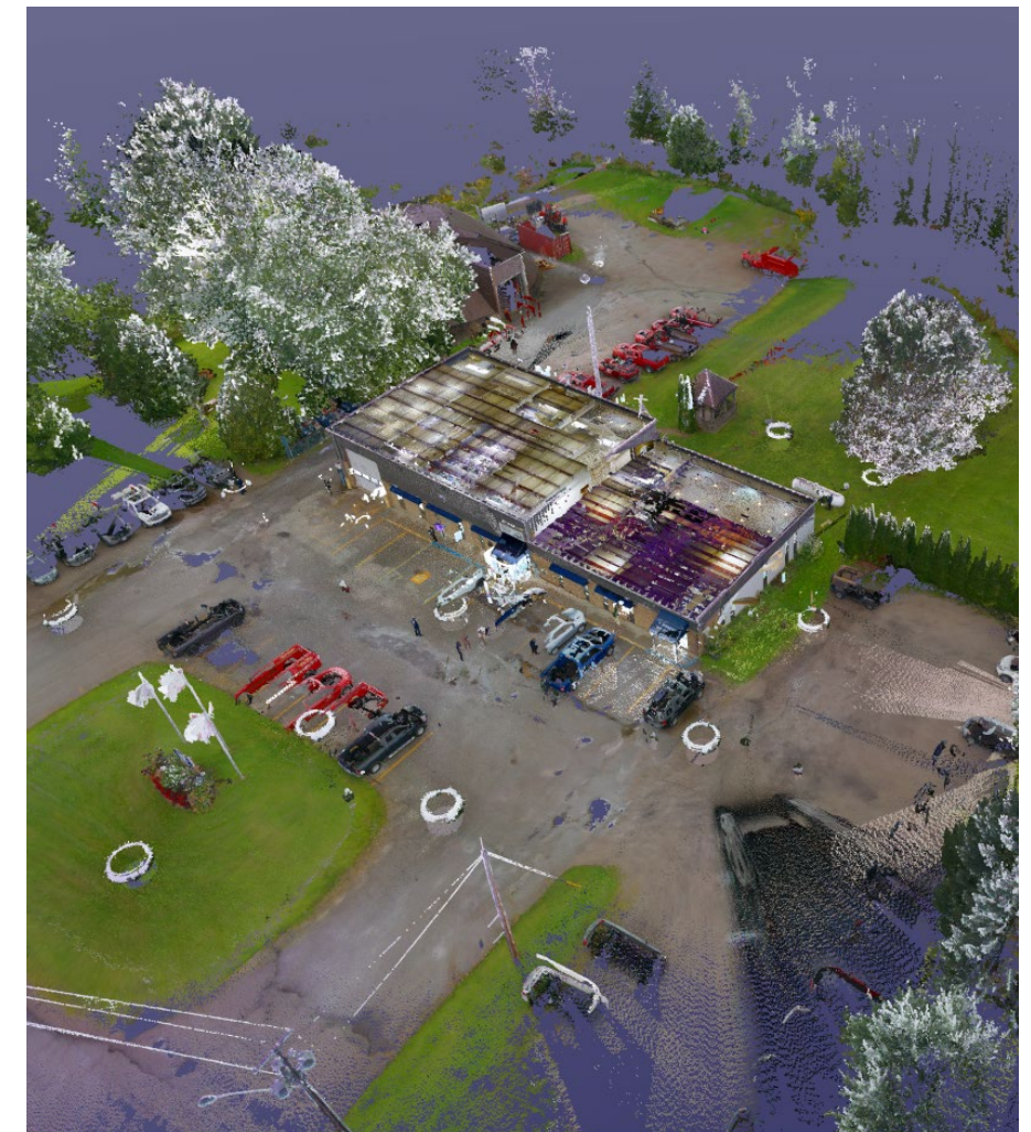
Existing Site Photographs
