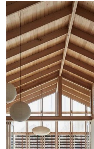
Council chambers ceiling
