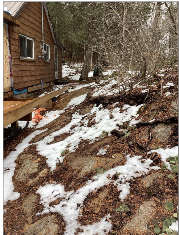
Photo 4 – Area along West Side Lot Line
