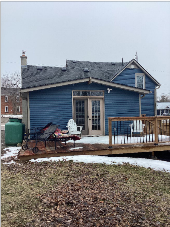
Photo 2 – Existing Constructed Addition
