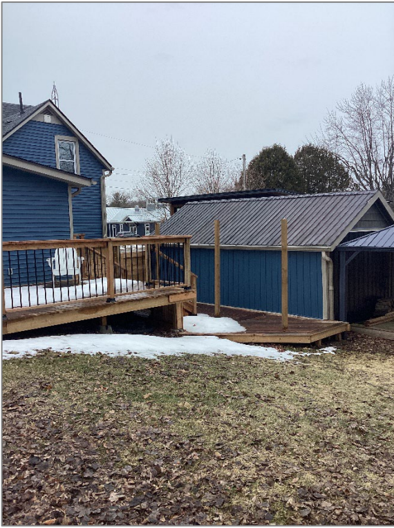
Photo 5 – Existing Deck to be Revised
