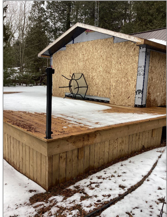
Photo 3 – Existing Deck to be Reconstructed and reduced in size
