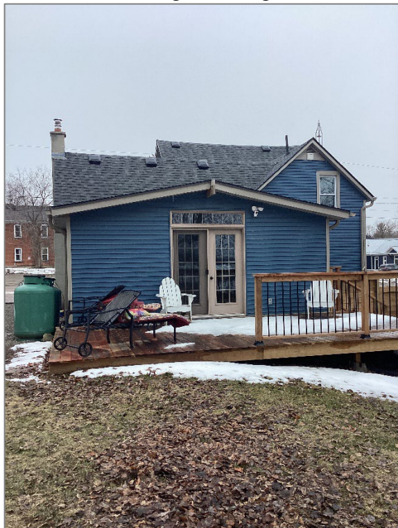
Photo 2 – Existing Constructed Addition
