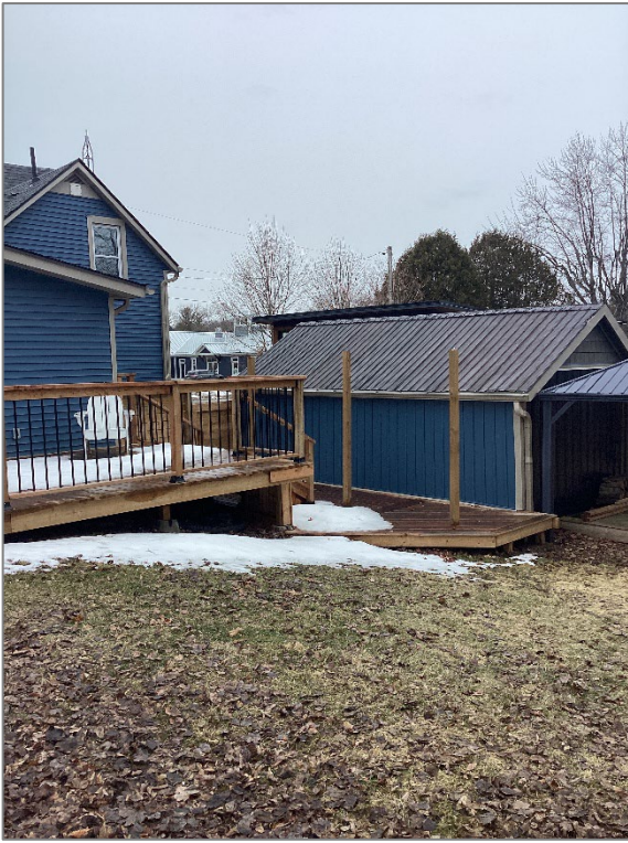
Photo 5 – Existing Deck to be Revised
